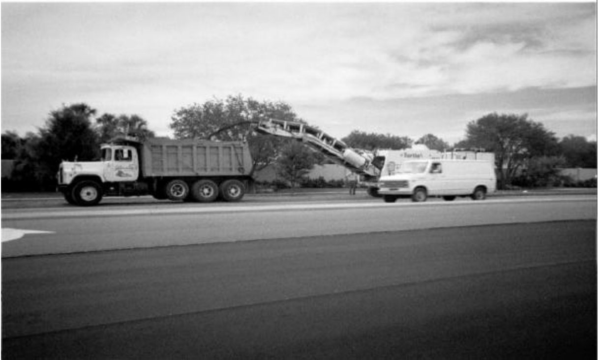
Figure 2.2 Typical Roadway Excavation Process
